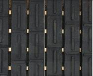
X-Lug flooring with open spacing between floor boards to avoid sewage congestion.
